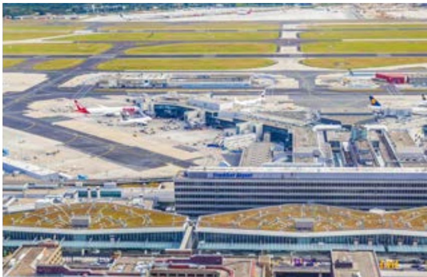
MTSC use case: Frank Airport, Germany
