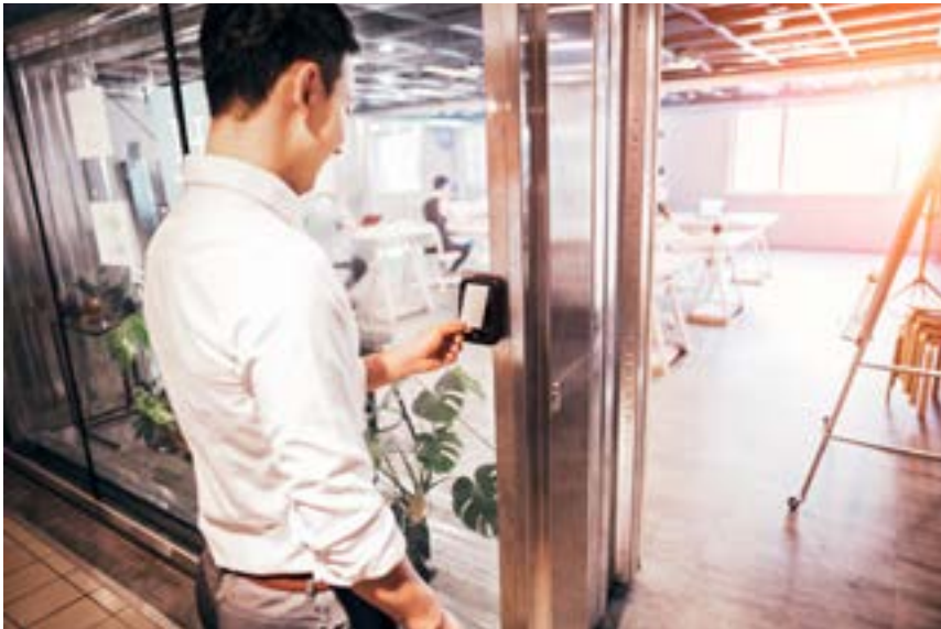
Access control systems can be compromised even before installation is completed
